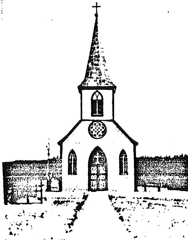
Fig. 5 Church at Fort Good Hope in 1933, showing new steeple and clapboarding.
